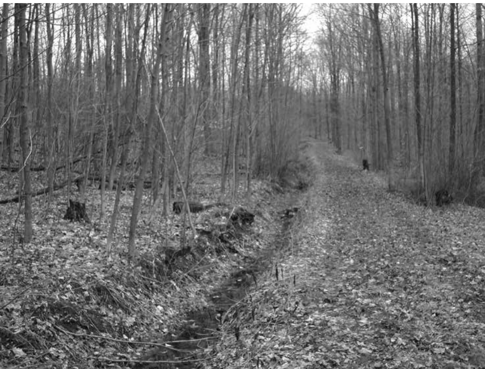
Figure 3. The owner of this road had a backhoe create a ditch on one side and pile the spoils onto the road. The road is now high and dry, serving needs for firewood, winter recreation and more.
