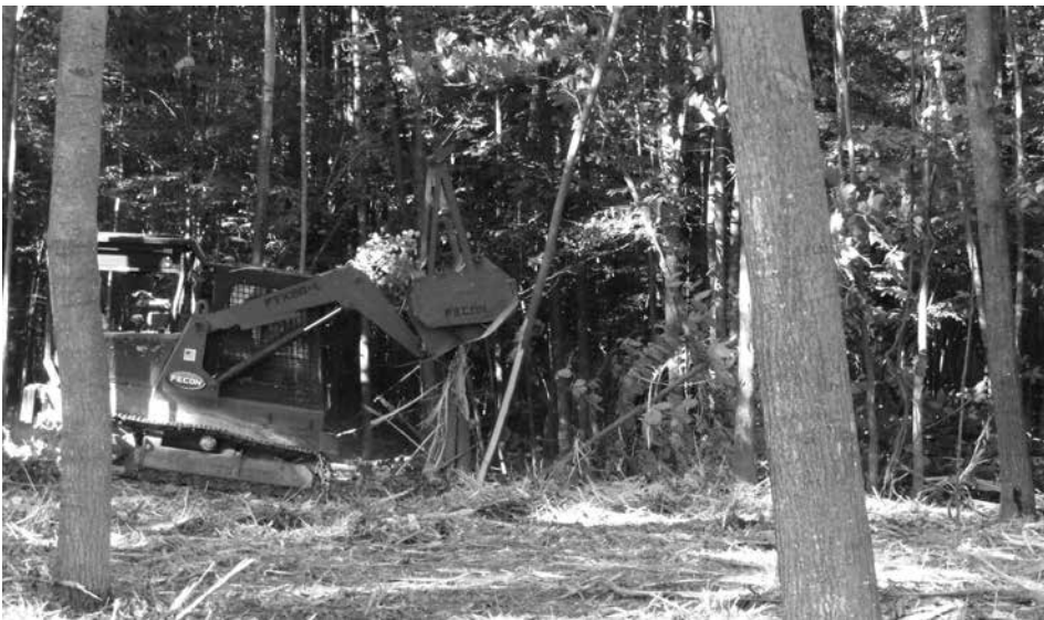
Figure 3. Purpose-built mowing machines like this FECON can reduce dense interfering understories to mulch. But before making this investment, consider what additional steps may be needed to prevent the freshly created void from quickly refilling with more of the same plants.
