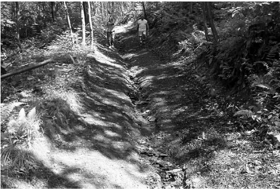
Figure 2. All trails have the potential for compacted and exposed soils. Without BMPs, water accumulates on the road from the canopy and via lateral flow on upslope positions, and the aggregate of water increases speed. The result is a trail with complicated access and the movement of soil to some other location.
