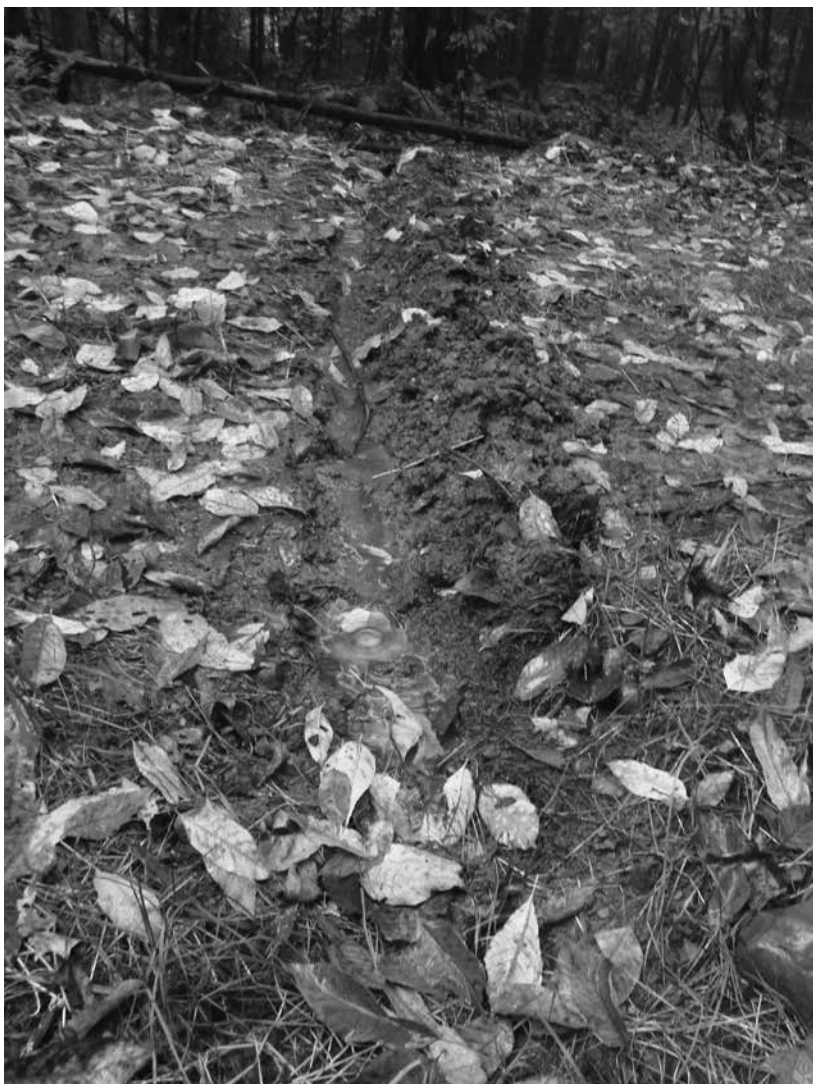
Figure 7. Appropriately scaled BMPs can provide the same benefit as BMPs used in commercial harvesting. This owner used micro water bars on an ATV trail. The water bars were effective and rebuilt as needed. Once vegetation was established on the trail, the need for these water bars diminished.
