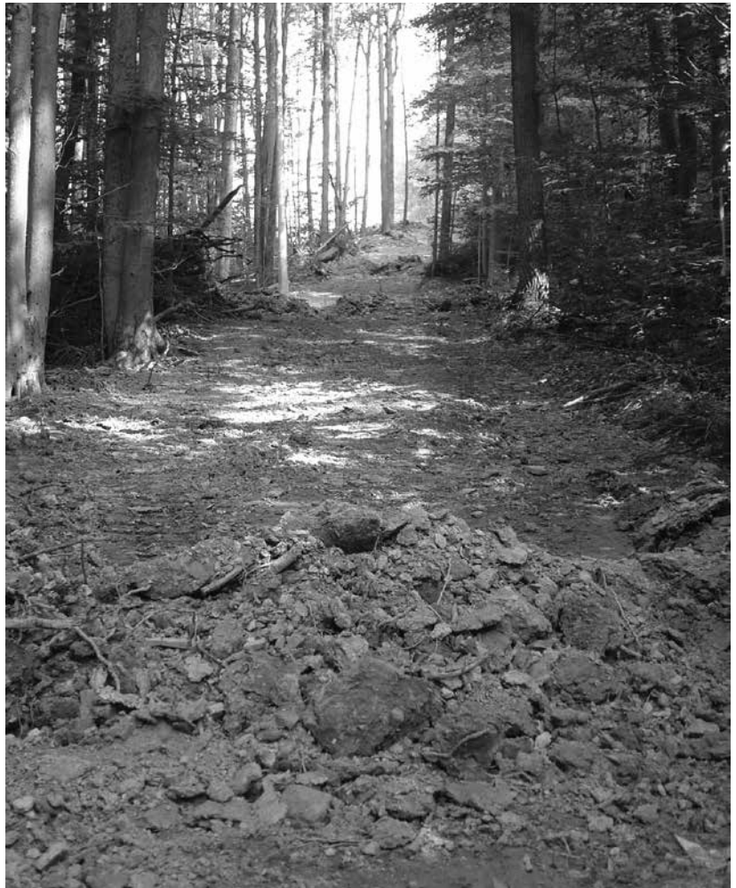
Figure 5. Water bars are an example of a water control structure. Water bars help manage water in small quantities and slow the movement of water. Water bar spacing is closer on steeper slopes, and the water bar is angled to deflect water off the road.
