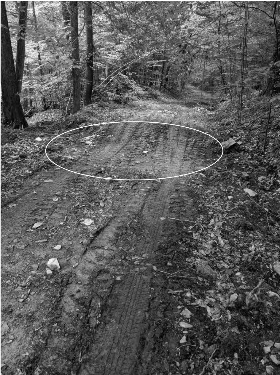
Figure 6. The circle marks the location of a broad-based dip on a limited access road. Broad-based dips provide a gentler reconfiguration of the trail or road than do water bars. The broad-based dip includes a berm that deflects the flow of water and are out-sloped to move the water off the road or trail.
