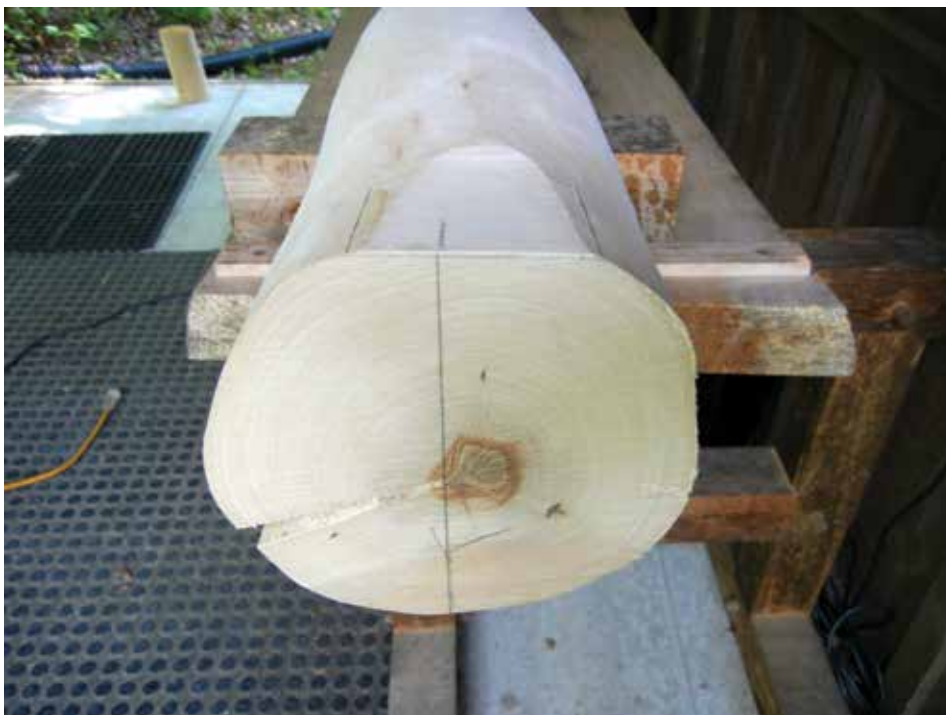
Figure 6. With the beam turned upside down, seat cuts were chiseled perpendicular to the end cuts to allow the pole to sit in a stable position without rolling once lifted into place.
