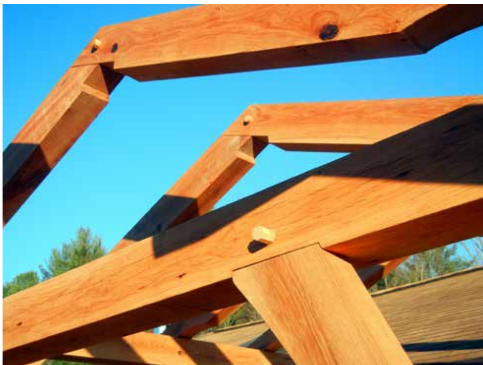
Figure 4. Its great structural strength combined with a high degree of rot resistance makes white oak a great choice for outdoor timber structures such as this porch in progress. Just be forewarned, freshly cut white oak is painfully heavy.
