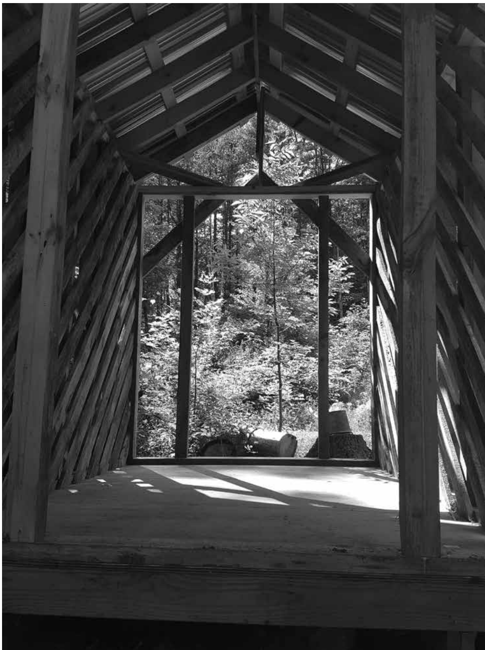
Figure 5. This woodshed is approximately 8 ft x 12 ft. The diagonal slats provide stability for the woodshed and a brace for each stack of wood that was stacked side to side. The metal roof had a 2 ft overhand allowing for storage of some tools on the outside wall.
