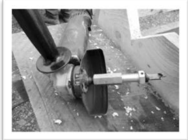
A simple work station made with notched lumber set on saw horses.
