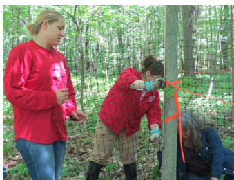
2"x 2" mesh fencing was installed 8' high to prevent the deer from entering the enclosed area.
