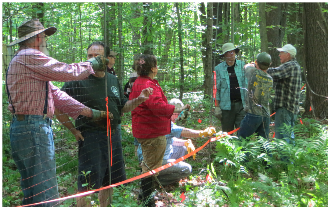
Rebar was used as uprights for the structure.
