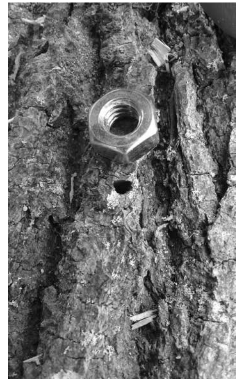
EAB emergence holes are about 1/8" in diameter and have a distinct "D" shape; 1/4" nut for scale.
