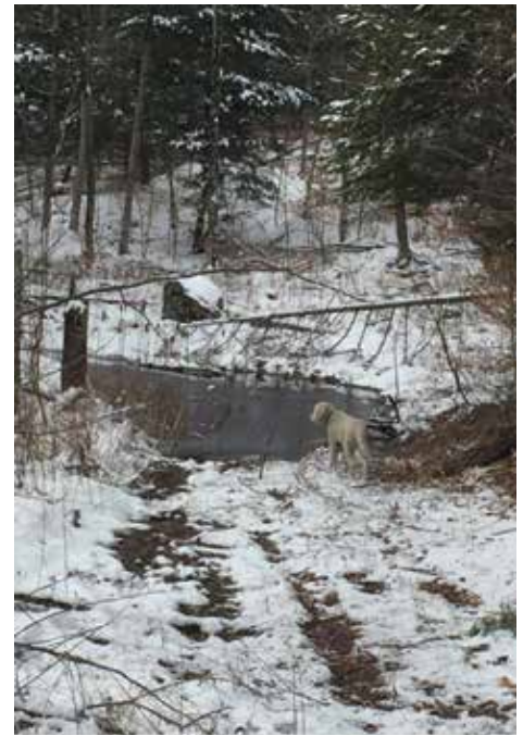
The access road to the upper tiers filled with water where the skidder from previous logging operations dug a hole going through the softer terrain. A new bridge is planned for this area.
