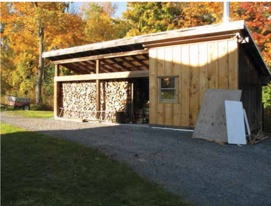
Firewood storage and Econoburn boiler room.
