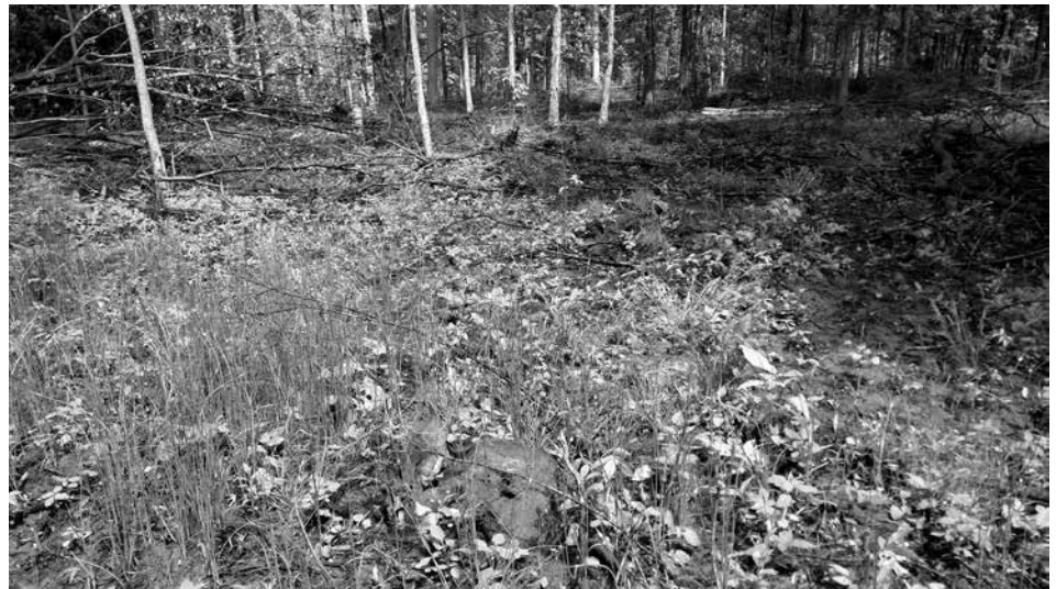
Figure 7. When clearing with a bulldozer be careful to keep the organic matter as intact as possible. The end result can be a clear and easily worked area. (Photo credit: Mike S.)
