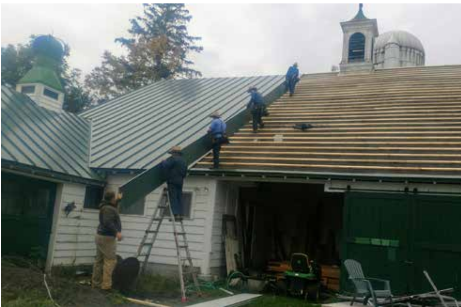
Renovation of the Cazenovia barn.
