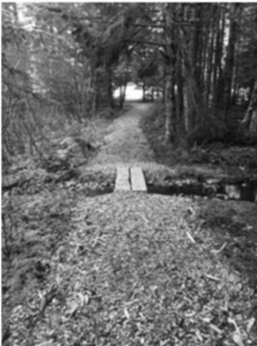
Completed & chip dressed recreational trail
