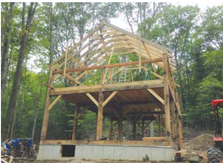
Barn raising in 2015 with red oak and other timber harvested on site.
