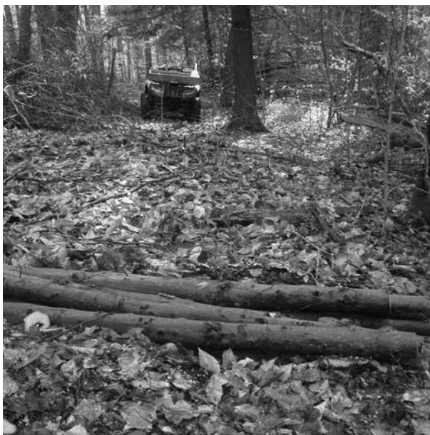
A corduroy base in a low spot in the trail reduces jarring of the machine and lessens impact and wear on the trail.
