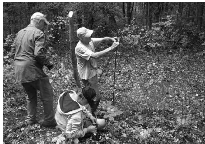
Attaching the fence to a steel rebar post.
