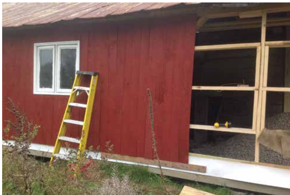
Rebuilding the barn with wood obtained from the property.
