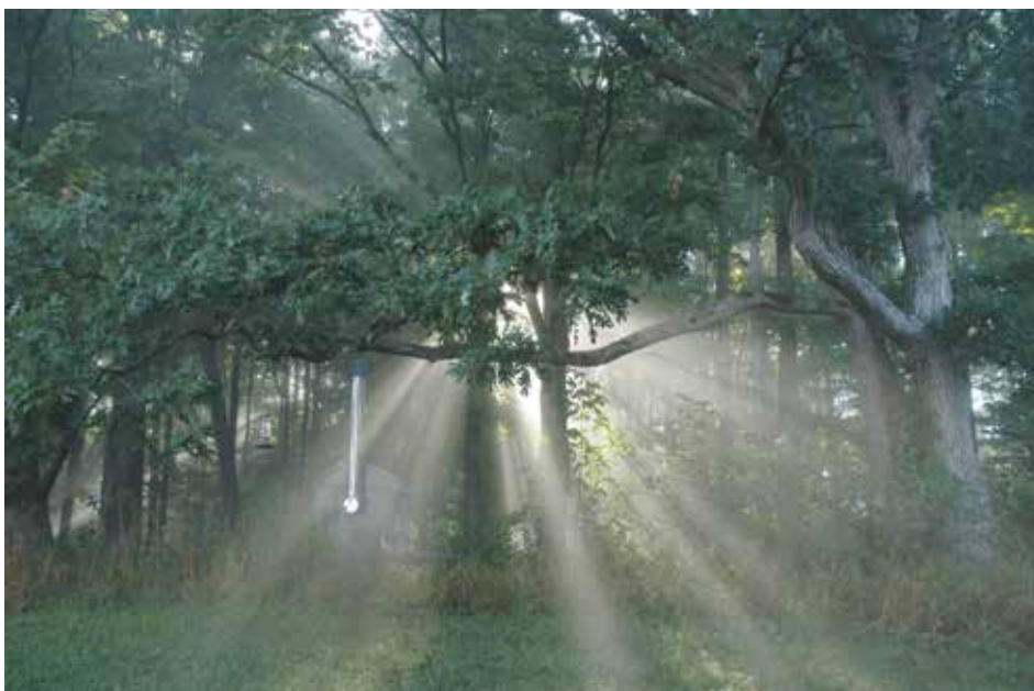
Outdoor wood boiler in a different light. Firewood from timber harvests and TSI work offsets 700-800 gallons of fuel oil.
