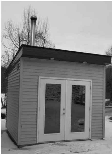
A 10' X 10' insulated shed provides plenty of room to shelter equipment, operator and about 40 bags of pellets, or a half a face cord of wood.
