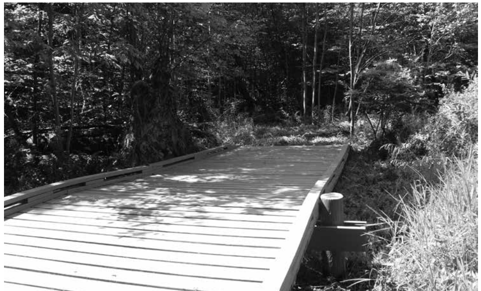
The Bridge to Nowhere two years after construction
