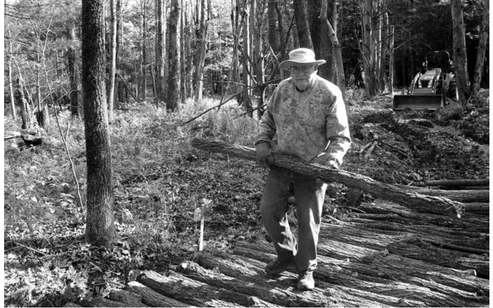
Tom Matteson working on a stretch of the corduroy.
