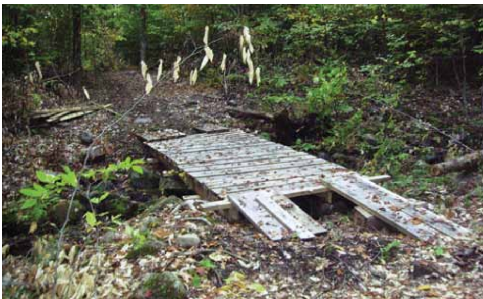
Larry Phillips built this bridge to access additional areas of his property with the tractor without disturbing natural water flows on the land.
