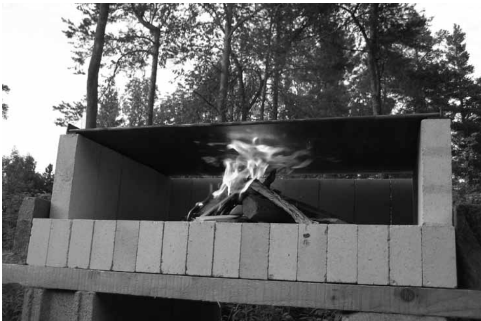
A simple, semi-portable brick oven with integral griddle that can be used to cook pizzas, breakfasts and lunches at the woodlot
