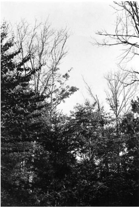
Figure 2. Sugar maple decline; crowns have progressively deteriorated, bark is sloughing off large branches and the upper boles.
