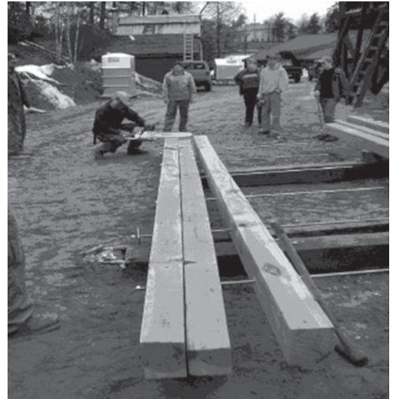
Angling the edge of a bridge cant with a chain saw.
