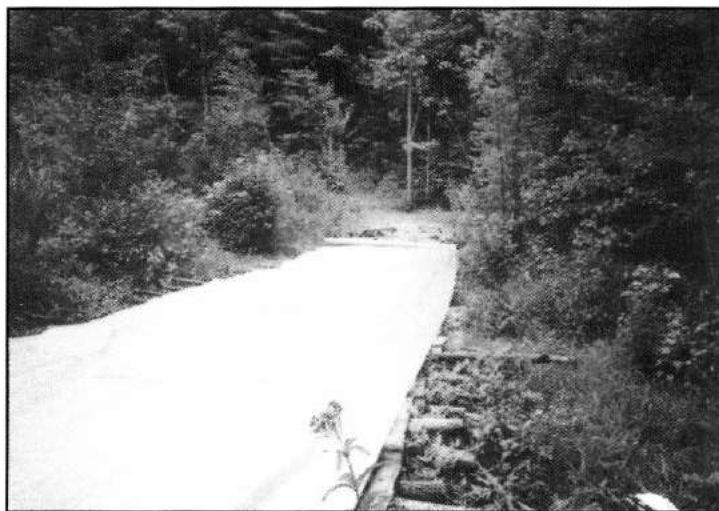
The spreading of the geotextile fabric over the log poles and pallets is seen during construction.
