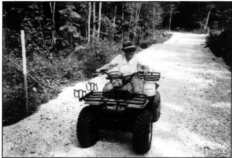
Late summer 1993. Robert Johnson drives his ATV on his newly completed access road.
