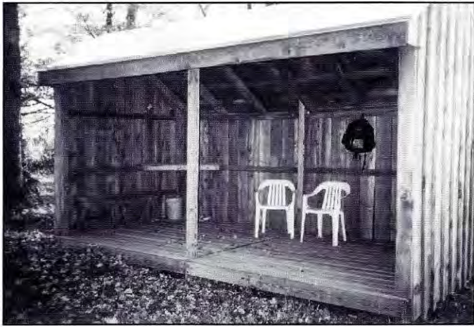
View inside the Wieder trail shelter
