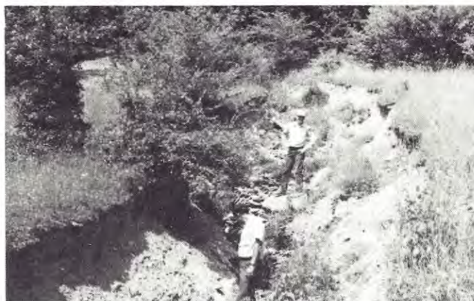
Right: Same road, downslope.
