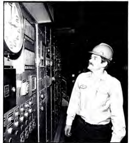
Dick McNamara checks the controls of the wood-fired boiler at Colgate University.
