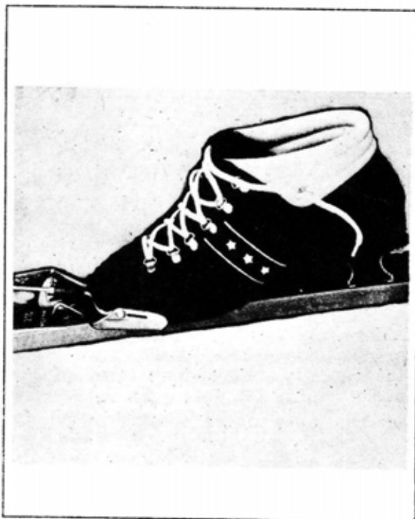
New type narrow ski with special boot and pin-and-clamp binding.
